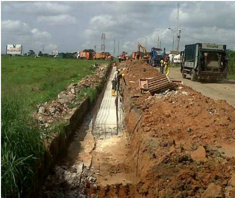
On-going construction of access road by Ministry of Works
