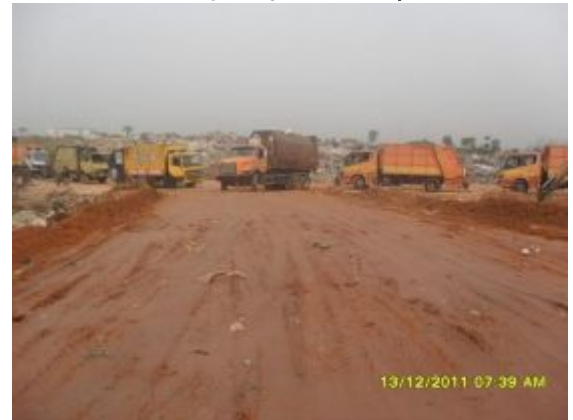
Road construction at Olushosun Landfill Site
