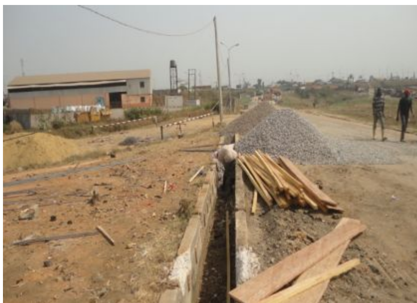
On-going road rehabilitation work at Olushosun Landfill Site
